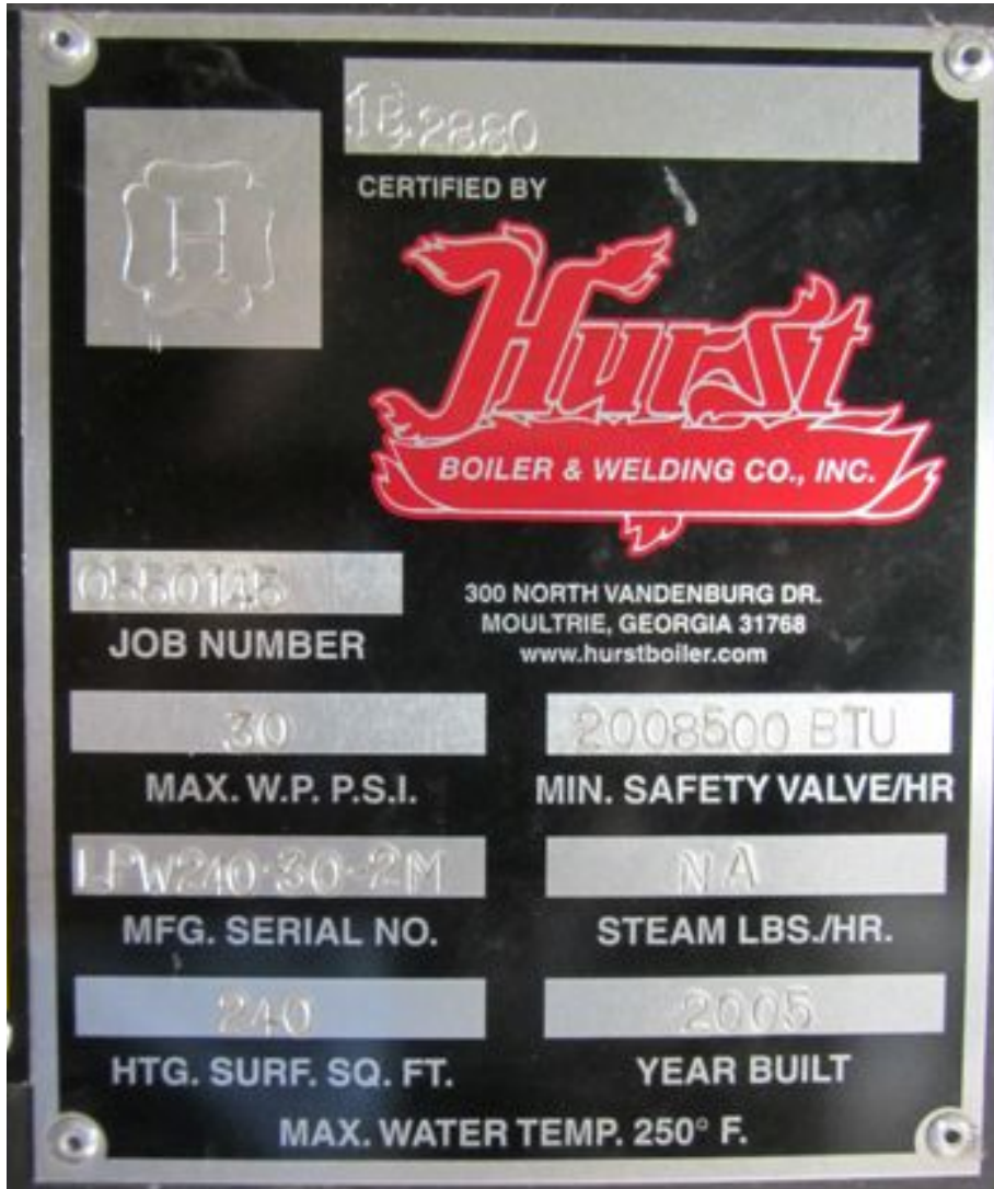
Photo 2. Nameplate for Hurst boiler
