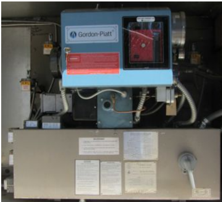
Photo 9. Gordon-Piatt burner on Workshop furnace
