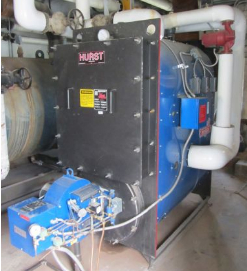
Photo 1. Hurst oil-fired boiler (2005)
