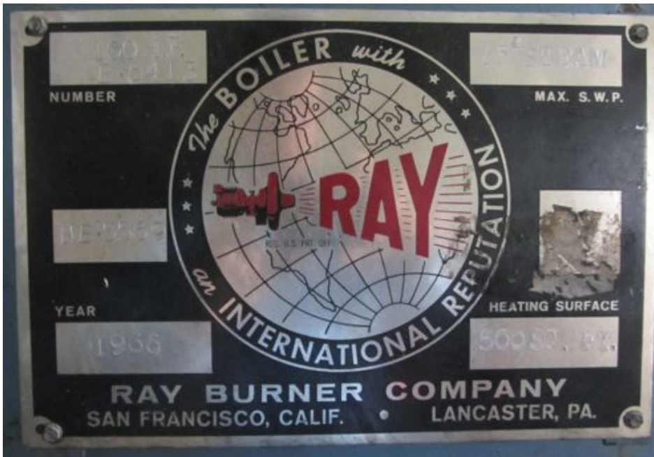
Photo 5. Nameplate for Ray boiler
