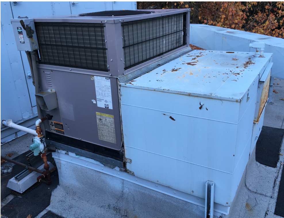
Photo 2 Bryant propane furnace on the rooftop of Plumas District Hospital.
