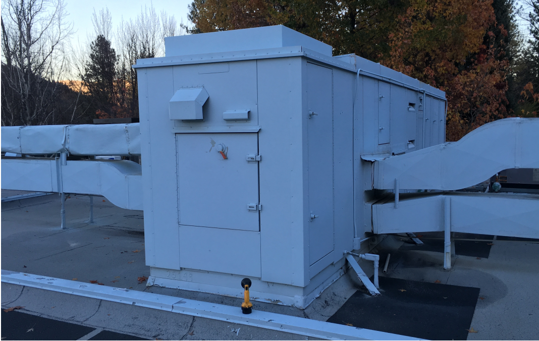
Photo 3 Propane furnace and air handler on the rooftop of Plumas District Hospital.
