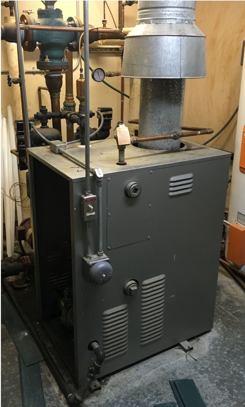
Photo 5 Bryan propane-fired hot water boiler in the Quincy Medical Building.
